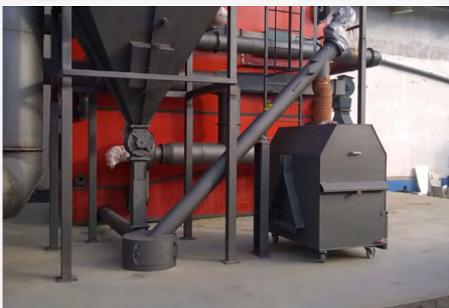
Automatic ash removal
