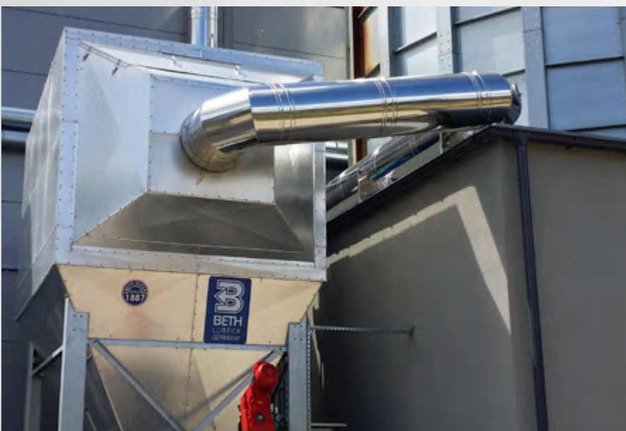
An flue gas electrostatic precipitator
