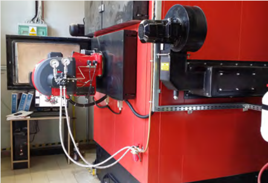
Burner supporting the combustion process
