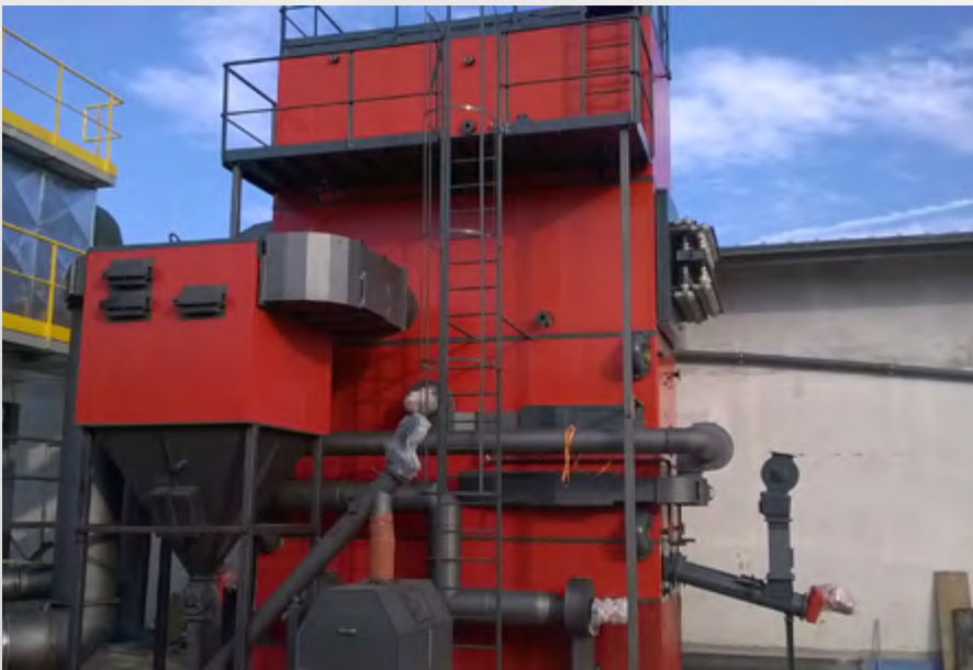
Steam boiler for agro pellets – 3 MW
