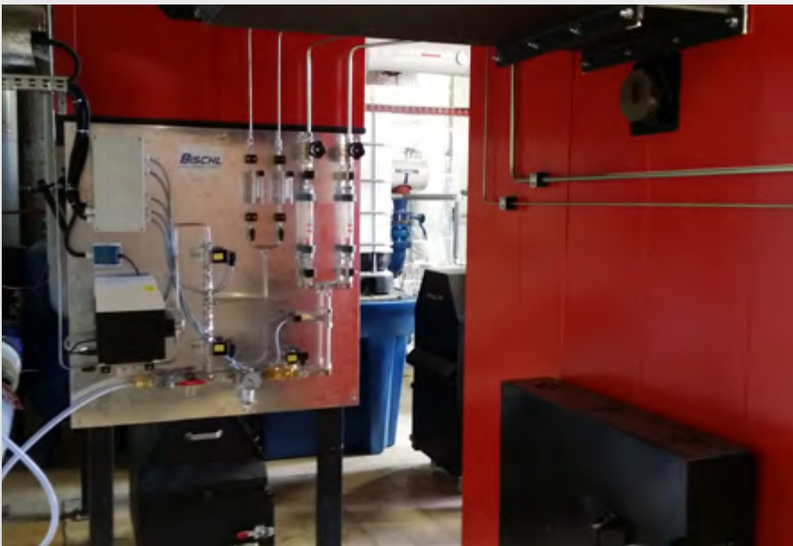
System NO x reduction - SNCR
