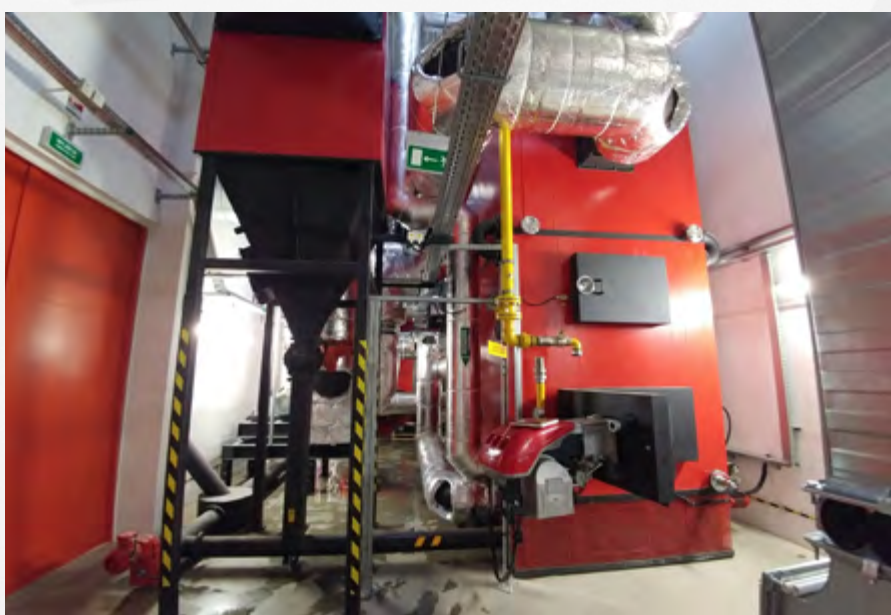
Boiler for wood waste – 3.3 MW
