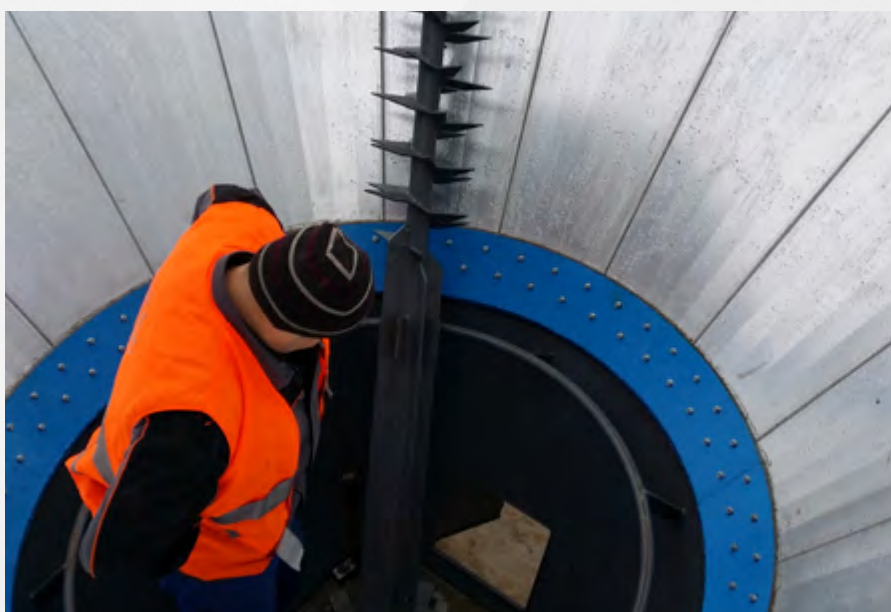
Oblique fuel scraper in silo
